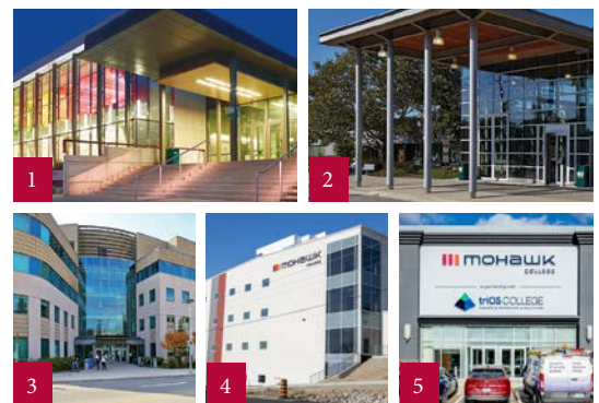
1. Fennell Campus, 2. Stoney Creek Campus for Skilled Trades, 3. Institute of Applied Health Sciences at McMaster, 4. Centre for Aviation Technology, 5. Mississauga Campus in partnership with triOS College
